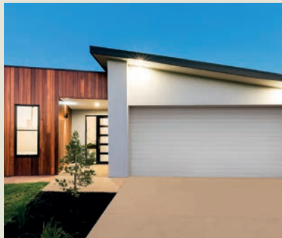
Abitazioni prefabbricate in CLS Prefabricated houses in CLS
